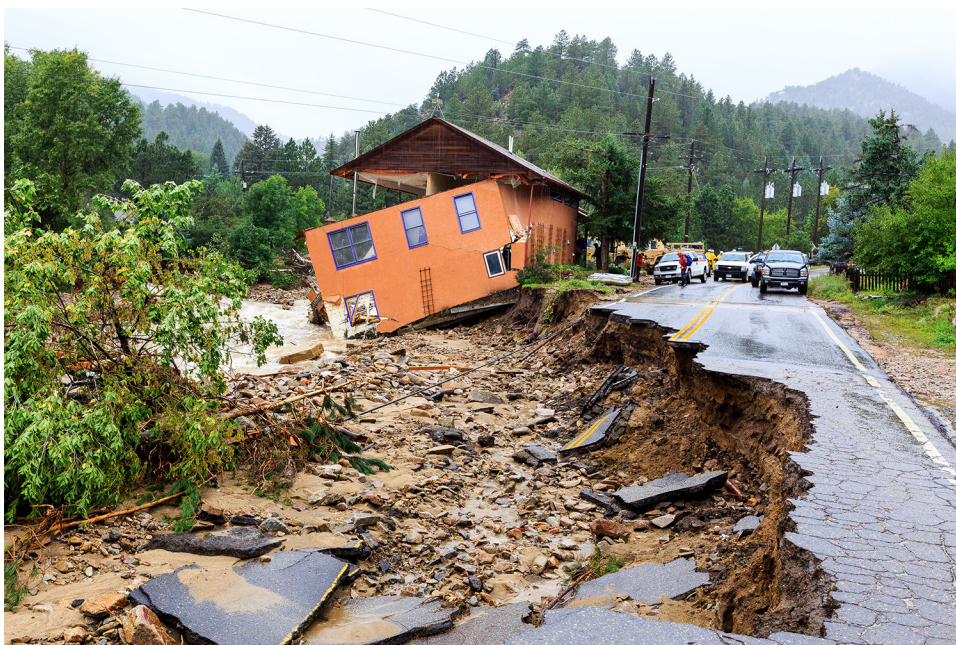
Damage from flash flooding in Colorado.
